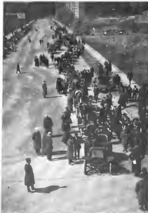
Starting at the Bottom of the Grade.
